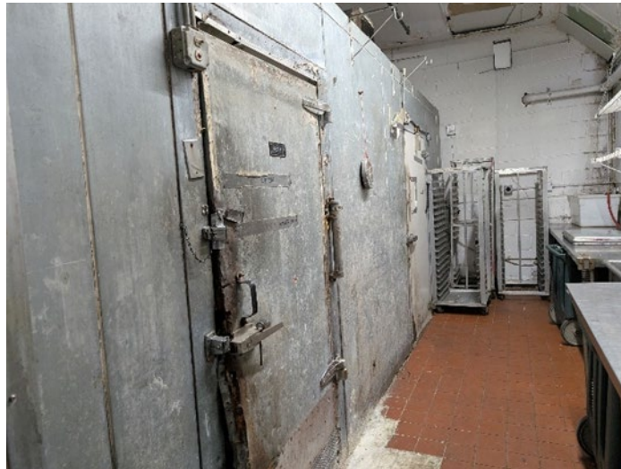
A view of a non-functional built-in deep freezer within the kitchen. The floor around the freezer has missing tiles.
