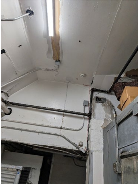
A view of the ceiling above the non-functional freezer pictured above. A hole in the ceiling is covered by a make-shift patch.
