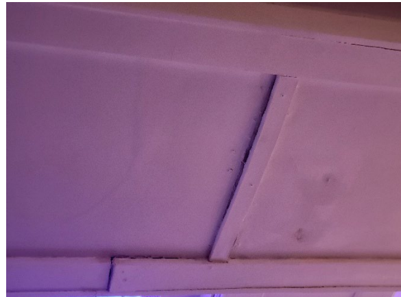
Above Left: View of the ceiling. Above Right: Closeup view of the ceiling in Gold Room where water damage from roof leakage has been patched and painted over.
