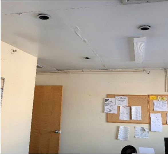
A view of warped drop ceiling tiles in an office (left). Another office space with patched ceiling and water stains from roof leaks (right).
