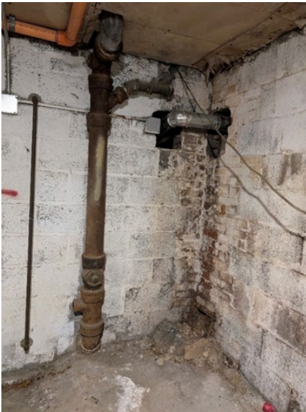
View of the corners in the basement hallways with exposed wiring as well as piled-up crumbling brick and concrete (above left and right).
