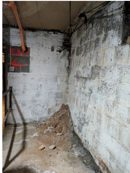
View of the corners in the basement hallways with exposed wiring as well as piled-up crumbling brick and concrete (above left and right).
