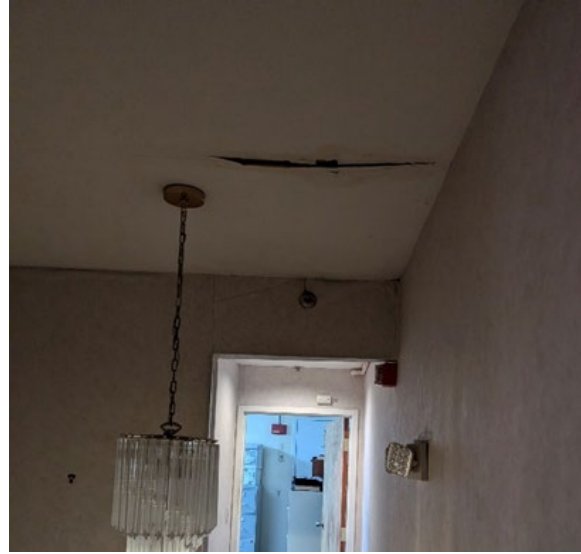
A view of the stairway leading from the ballrooms on the ground floor to the offices at the upper level (left). A close-up view of the water damage from the leaking roof can be seen (right).
