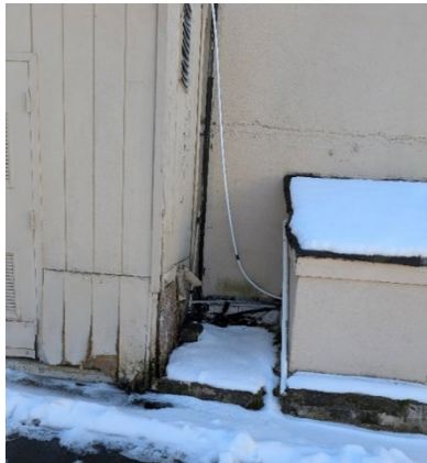
Above Left: A closeup view depicting the rotting wood and damage at the base of the utility shed storing the high voltage equipment. Above Right: A closeup view of the narrow drive-aisle that connects the two sections of the rear parking lot. The drive aisle exhibits significant wear and tear with large cracks and potholes. Also pictured is the fence-screening the trash compactor and outdoor storage/loading area from Claremont Avenue.
