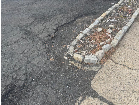
As seen in the above pictures, the parking lot is ill maintained with potholes and lack of defined parking spaces.
