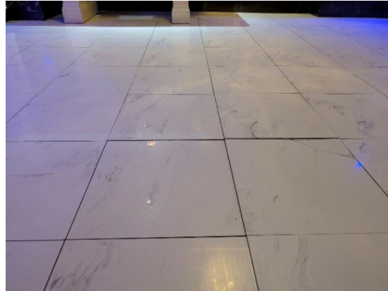
View of the lounge on lower level (below ballrooms). As reported by the property owner, the uneven tiles are due to uplift from water infiltration and frequent repairs.
