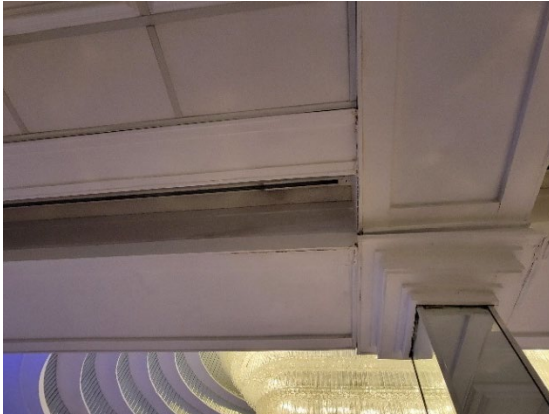
A view of the ceiling and pillar in Regency Room showing warping and water damage from roof leaks that have been painted over to hide it.
