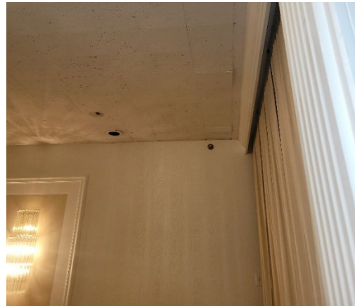
A closeup of the warped drop ceiling tile in the chapel on ground floor of building. Although frequently patched, as per the property owner, water infiltration is also an issue in this room.
