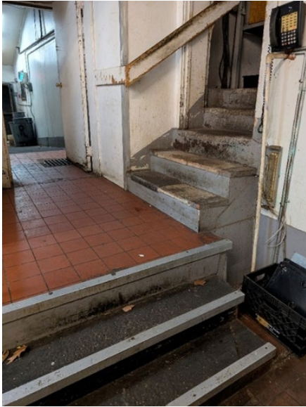
A view of the staircase leading from the kitchen to the upper level. Stairs are missing tiles and show significant wear and tear.
