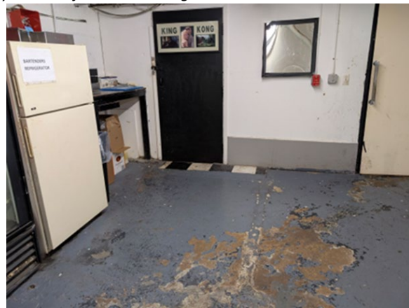
A view of the kitchen space with bartender's refrigerator exhibiting wear and tear on the concrete flooring.
