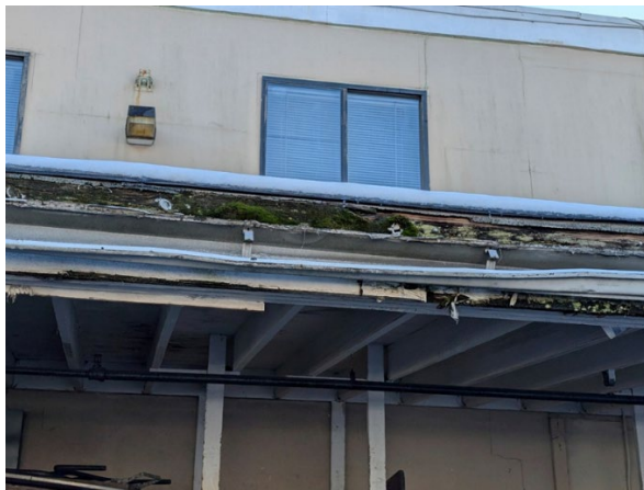
Above Left: Close-up view of the roof above the storage and loading area. There is missing siding, and the gutters are partially detached.
