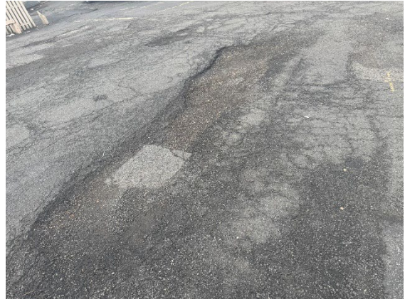
As seen in the above pictures, the parking lot is ill maintained with potholes and lack of defined parking spaces.
