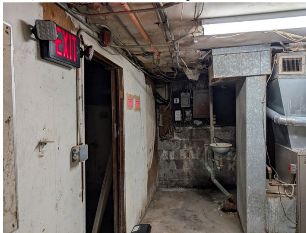
Pictured above is the entrance to a storage room in the basement. Peeling and warped ceiling tiles, water staining, exposed wiring, and aging plumbing indicate obsolescence and lack of maintenance.
