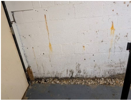
Above Left: View of the basement floor. The gap between the foundation and concrete floor in this area is filled with stones and dirt.
