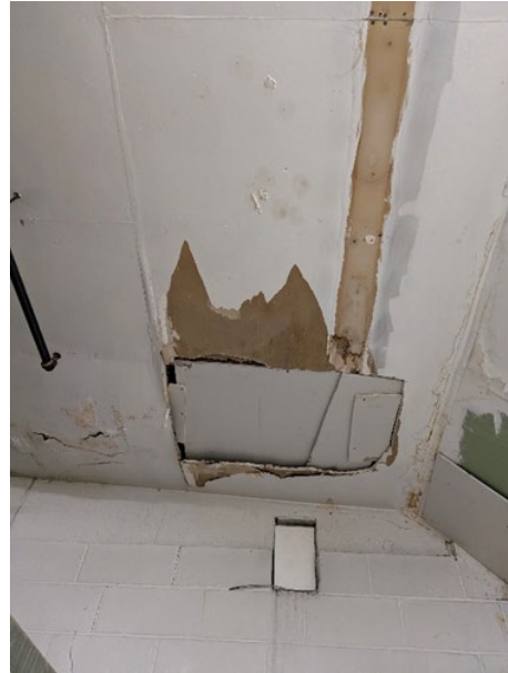
A view of the ceiling above the non-functional freezer pictured above. A hole in the ceiling is covered by a make-shift patch.
