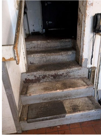
A view of the staircase leading from the kitchen to the upper level. Stairs are missing tiles and show significant wear and tear.
