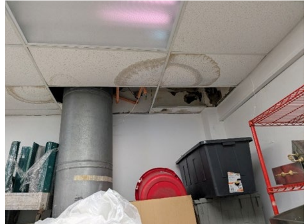
Above Left: Another view of ground floor storage area. Above Right: A closeup view of the ceiling in the ground floor storage area with missing tiles. Water stains show water damage probably from roof leakage.
