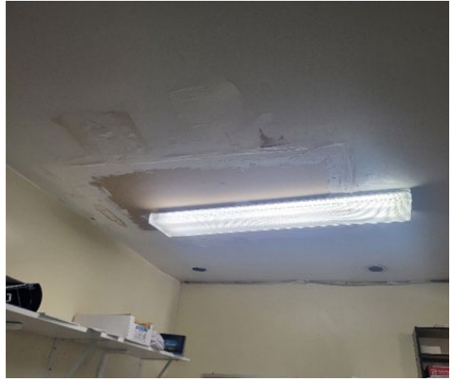
A view of warped drop ceiling tiles in an office (left). Another office space with patched ceiling and water stains from roof leaks (right).
