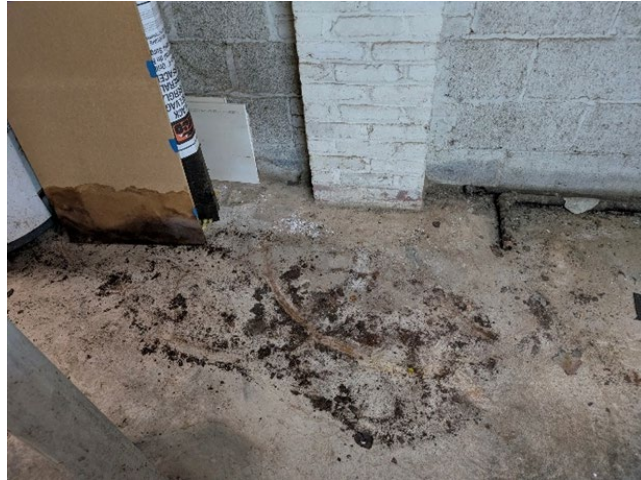
Above Left: View of rough, patchwork repair on the ceiling in the basement. Above Right: In addition to a large hole and exposed wiring, this area exhibits staining and possible mold from water infiltration. Also pictured (below left), in a separate area within the basement, water stains along at the base of the walls which are indicative of water infiltration.
