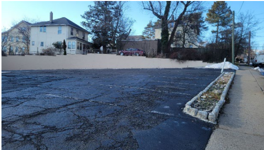
Above Left: Rear Parking lot (northeasterly side of building). Also pictured are two points of ingress and egress onto Claremont Avenue. Parking lot has cracked asphalt and undefined parking spaces.
