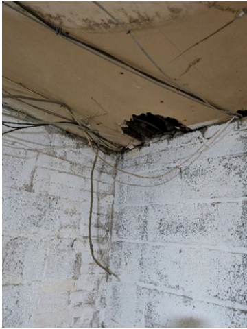
Above Left: View of rough, patchwork repair on the ceiling in the basement. Above Right: In addition to a large hole and exposed wiring, this area exhibits staining and possible mold from water infiltration. Also pictured (below left), in a separate area within the basement, water stains along at the base of the walls which are indicative of water infiltration.
