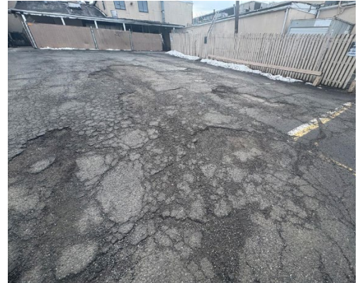
Above Left and Right: Another view of the parking lot in the northwesterly section of the property. No clear signage for parking or loading areas is visible. The parking lot is in a state of disrepair.
