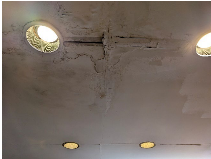
Water damage from the leaking roof is more evident in the offices that are on the upper floor. Seen above is water damage and warped ceiling tiles in the main office.
